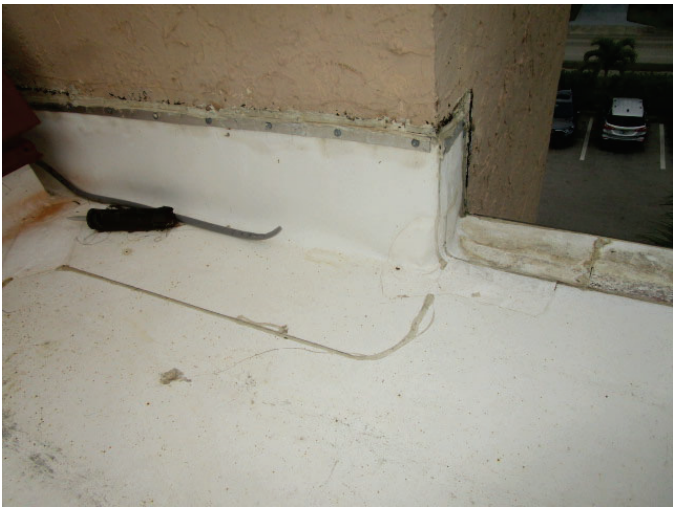
Roof covering: 2019 TPO vinyl main "flat" roof
