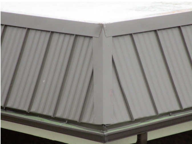
roof covering: 2019 Metal mansard
