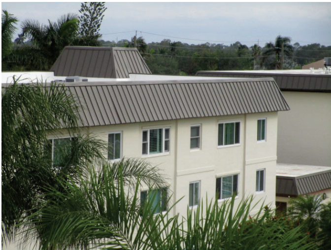
roof geometry- Flat w/mansard
