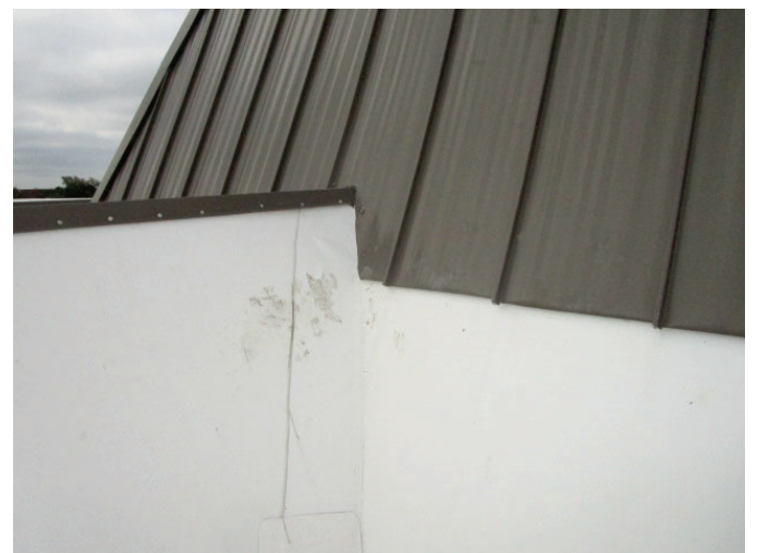
2019 TPO vinyl flat roof w/2019 Metal mansard
