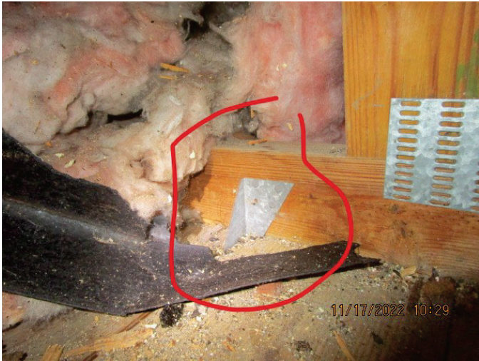
roof to wall attachment: hurricane clips
