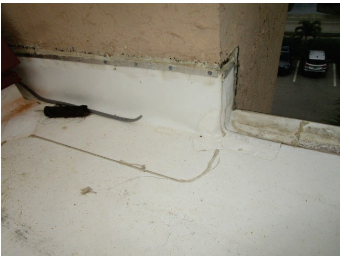
Roof covering: 2020 TPO vinyl main "flat" roof
